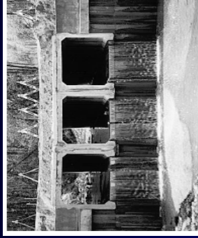
Figure 1-5--Precast Concrete Box Culvert (American Concrete Pipe Association)
